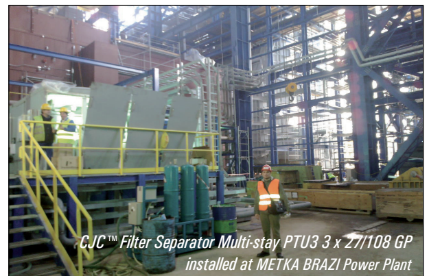
METKA BRAZI Power Plant, Romania
